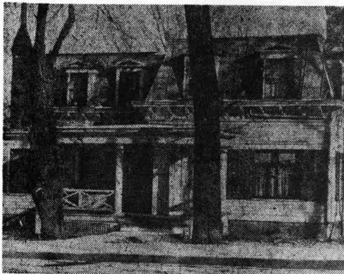
Britton Residence Built Solidly by Squire Beach-- Original Work Lasts
