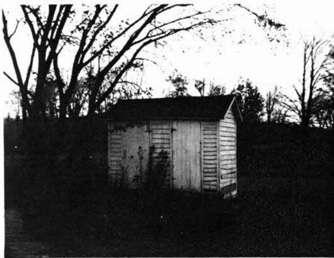
Behind the country school, the "necessary." Osborneville district school on Rock Island Road, one of many deserted buildings of a forgotten era.
