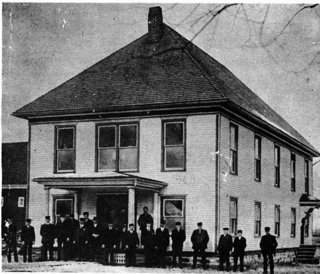
Pictured above is the home of Crary Mills Grange. The Grange itself was founded on January 20, 1874, but it got around to building the Grange Hall only during the Summer of 1905. The building pictured is only part of today's Grange Hall because it underwent "surgery" after it was built and proved too small. At that time, carpenters sawed it in two, right in the center. The two halves were shoved apart and a new segment was built between them. Few if any of the Grange members, all residents of the Crary Mills area, pictured in the photo are alive today.
