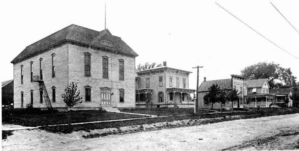
Hammond Advertiser is building third from left (town hall which burned). Building now a plumbing shop.
