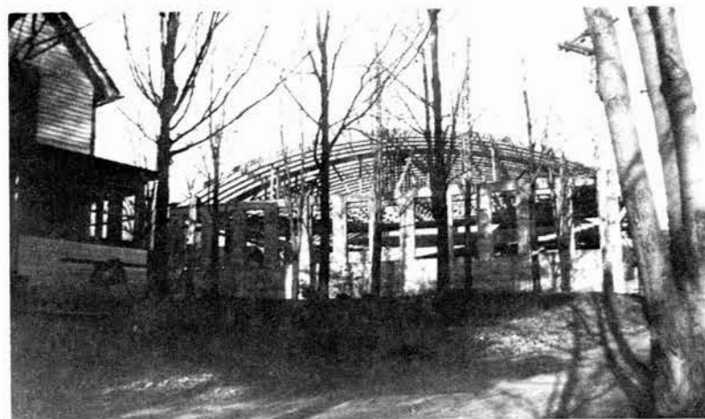
Building a part of the Kerr Garage which collapsed in February 1971.
