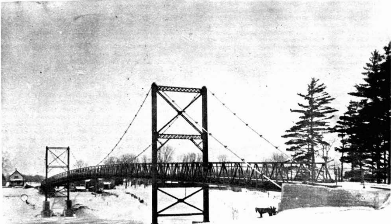
Massena Center Suspension Bridge. Picture taken in January 1911. Designed and built by Holton D. Robinson in 1910, his first bridge. Span 400 feet across the Grass
