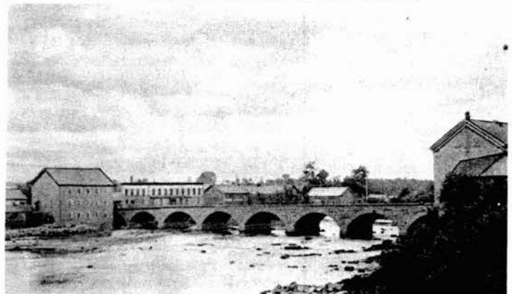
A Johnson Stone Arch bridge at Madrid built in 1889.
