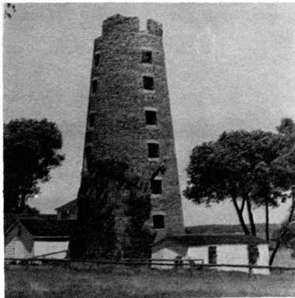
The Prescott windmill is 28 feet in diameter at the base, and the stone walls are 58 feet high. There are four columns
