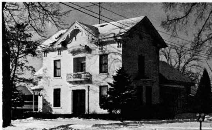
ITALIANATE WITH VARIATIONS, 16 Elm St., Potsdam. Built in 1863 by John Pert, is now the residence and office of Dr. E. S. Prescott. This shows a combination of styles in this period. Tour was designed to instruct in recognizing different styles.
