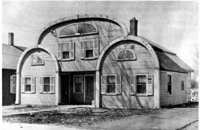
Royal Arch Mason House, built by Paul Boynton about 1856 at 12 Pine St., Canton.
