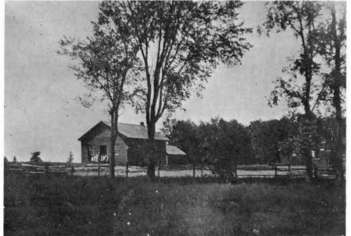
Red Brick School at Brasher Center
