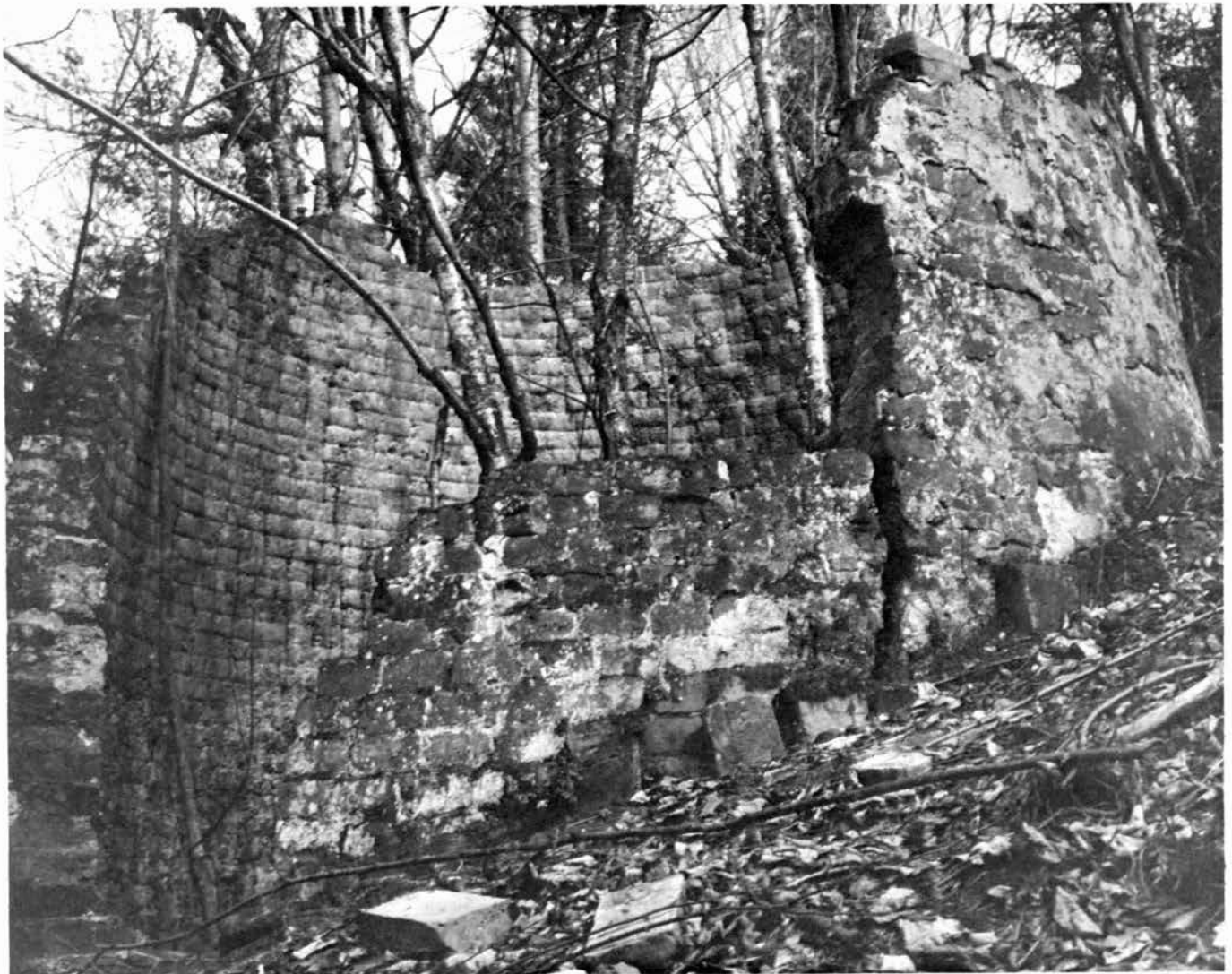
Ruins of the old Myers Steel Works at the abandoned village of Clarksboro, where ore was smelted into pig iron, thence shipped to East DeKalb over the old wooden railroad, (Jack Thomas Photo)
