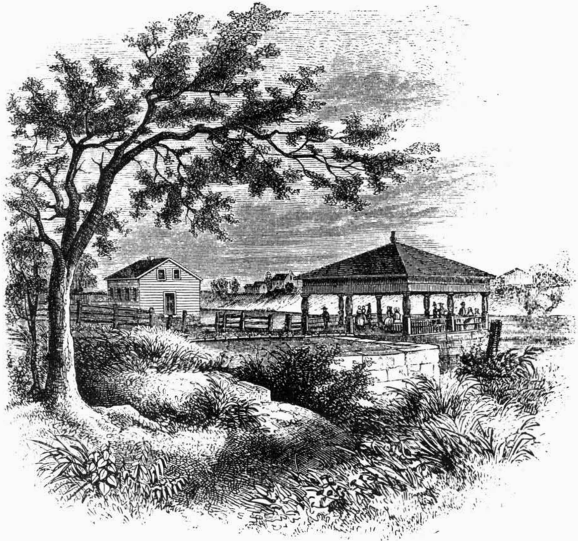
THE SPRING, AND THE BATH-HOUSE, MASSENA SPRINGS.
