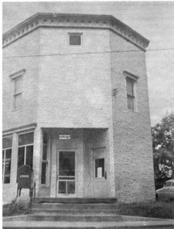
Post office in first floor of Masonic Hall, Edwards. Its unusual sculptured metal architecture is painted aluminum.
