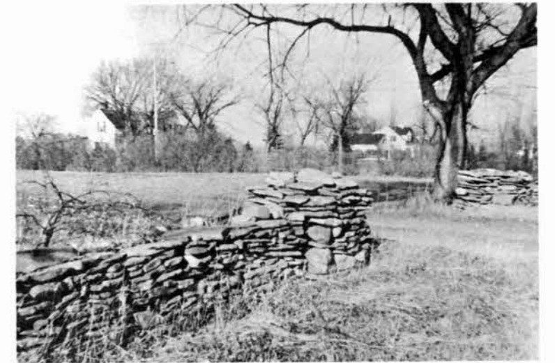
Flat stones laid without mortar (Town of Oswegatchie).
