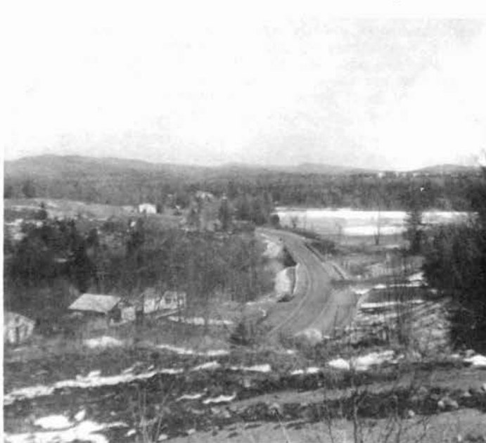
Upper Hudson River Bridge in Spring of 1967.
