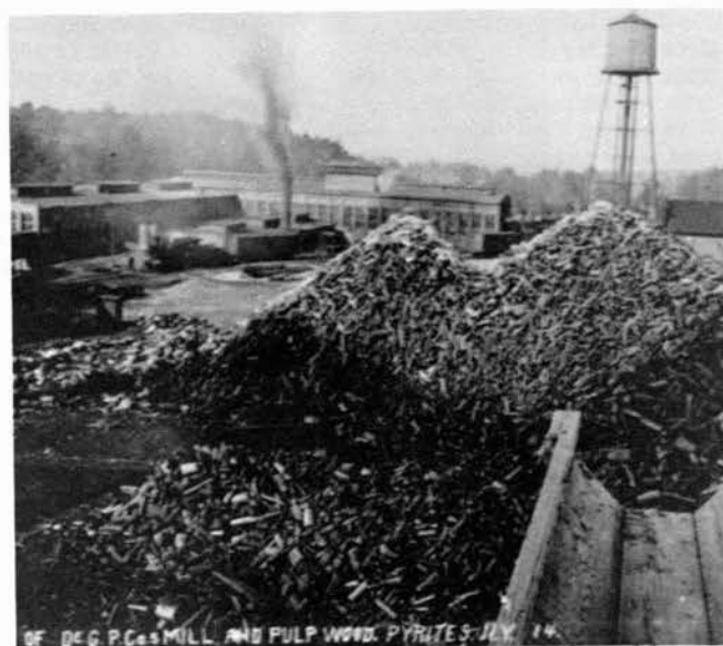
Front view of mill, taken from log chute.
