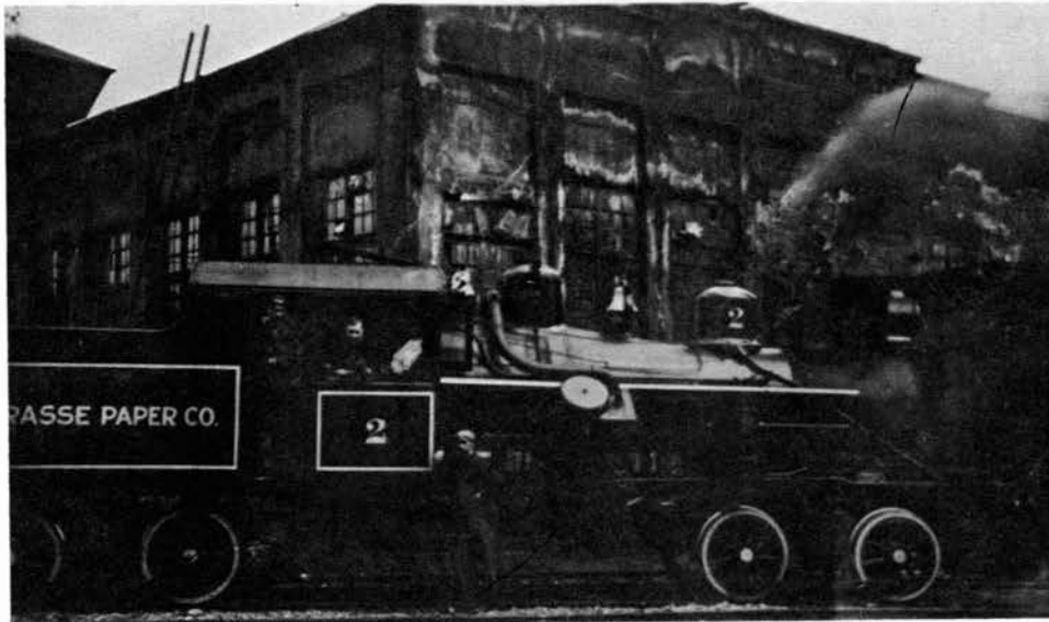
Locomotive back of papermachine room
