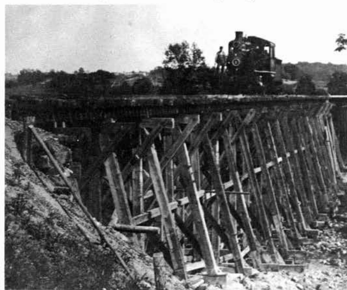
Switch engine on trestle
