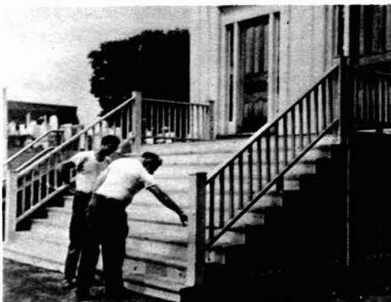
Putting the finishing touches on the new steps.
