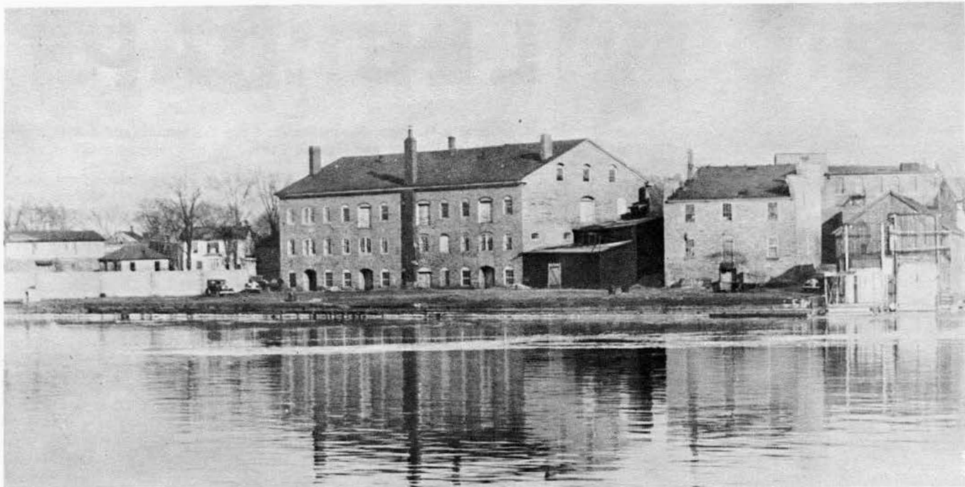
THE BUILDING AS IT APPEARED IN 1936
