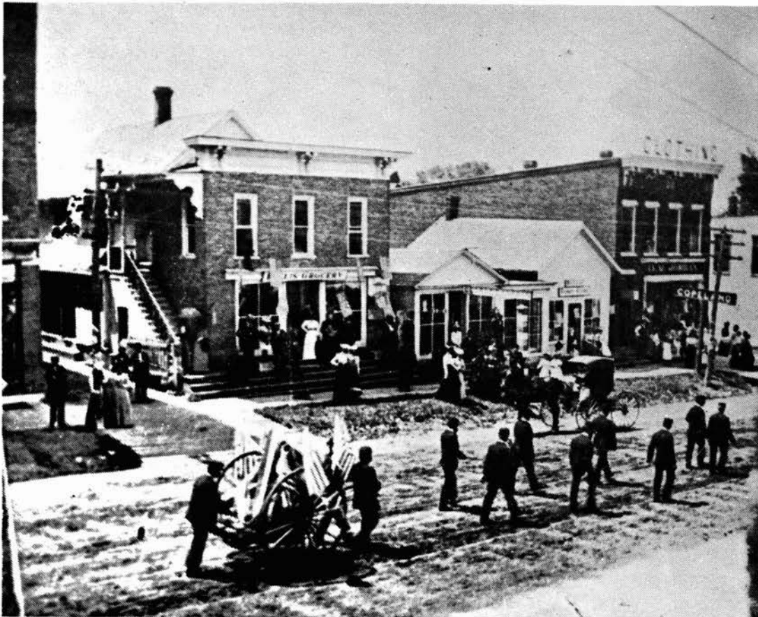
Canton Main Street at the turn of the Century, showing the site of the present First National Bank building.
