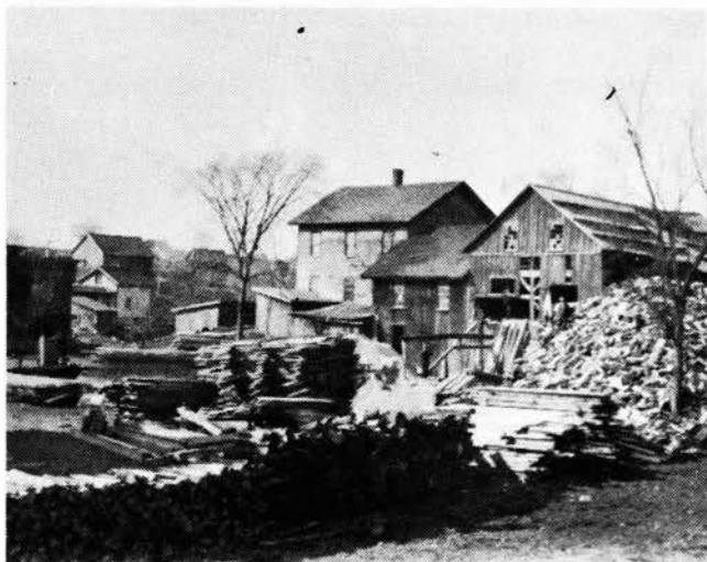
Pope's Sawmill and Gristmill run by the Pope Family from 1816 to 1927. Note Grange Hall in left background (Photo from County Historian's Collection)
