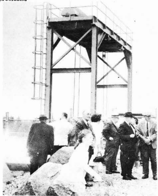
STARK POWER STATION
